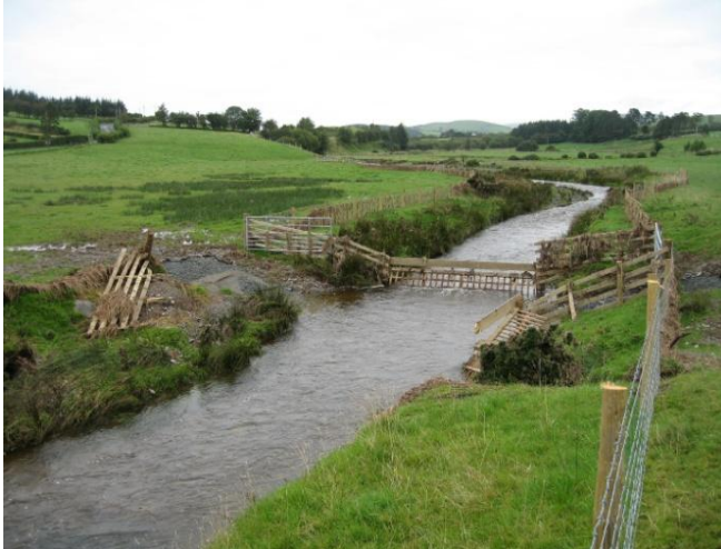
Fig 4 Post September 2008 flood
