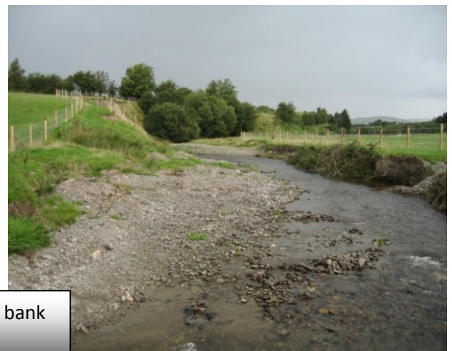
Fig 2 Pre-works condition of Afon Marteg
