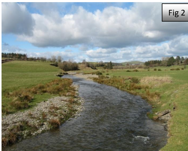
Fig 3 Soon after initial works completed. Note, double bank fencing and soft revetment of erosion prone bank
