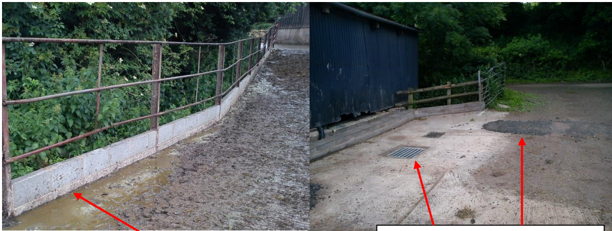
New cross drain and dirty water tank intercepting yard run-off- previously discharging into the watercourse
